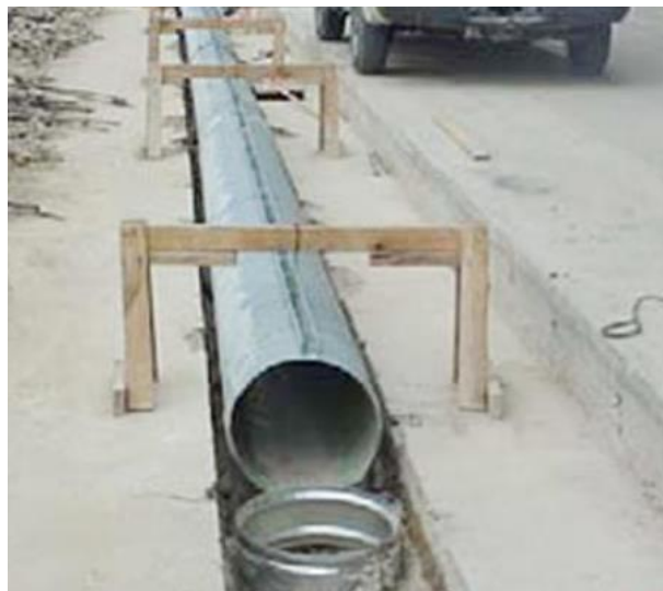
Figure 6: Corrugated Metal Pipe Storm drain [6]
