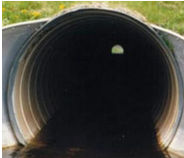
Figure 9: 48” Corrugated Metal Pipe Storm drain to be used in parking lot [6]
